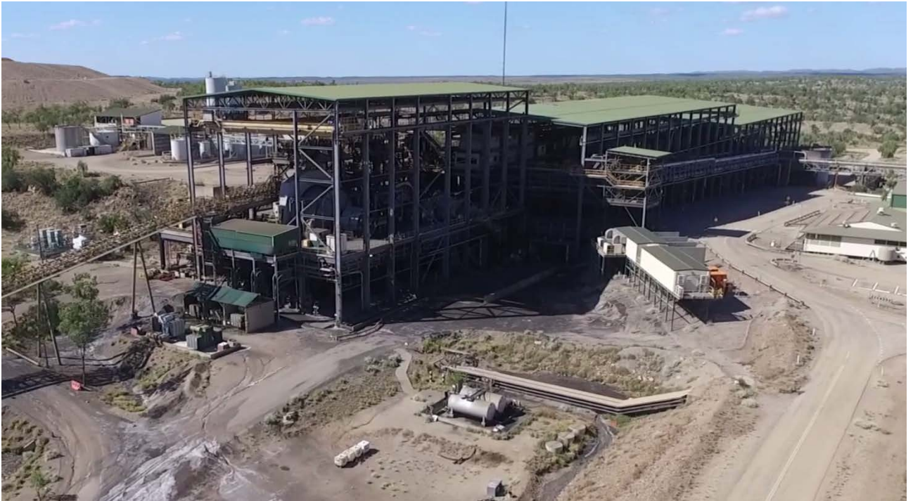
The Century Processing Plant
