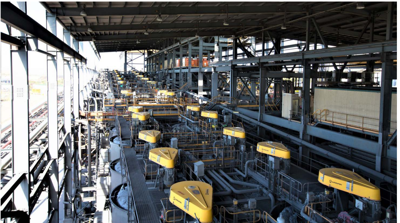
The Century Processing Plant
